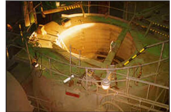
Installed rotor inside stator
